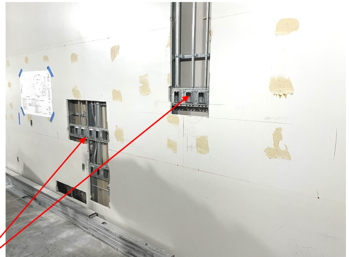
The top-right photo shows the last of the electrical infrastructure that needed to be installed in the west wall of the future Student Government Room. Here you can see all of the necessary electrical and A/V support that will power the future flat panel tv and connected computer in this area.
