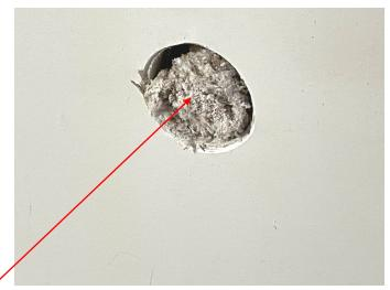
The top-right photo shows the evidence of the new blown-in cellulose insulation that was installed in the stud cavities in the existing wall between the future Student Government Room and the existing Data Processing Office Suite next door.
