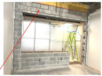
All three photos show the work that was accomplished this past week which was basically a lot of masonry detailing. After the new steel support lintels were installed last week this allowed the masons to fill in above and around the new window and entry systems with concrete block that will eventually be covered by new furring strips and wallboard.
