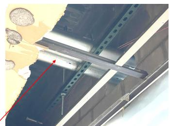
The top-right photo shows some the new conduits that were installed in the corridor that will convey new electrical wiring and data cabling into the project areas.
