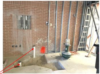
The top-right photo shows the completed rough plumbing installation. The two pvc pipes shown are for drainage of the sink and toilet that will be installed towards the end of the project in the future single-occupant (unisex) restroom.
