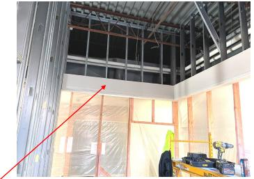
The top-right photo shows the new bulkhead in place that will help transition the new ceiling in this area into the existing. This bulkhead is needed because the existing spline ceiling tile system is no longer being produced or used and now a suspended acoustical tile ceiling system will installed instead.
