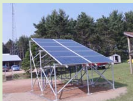
A charging station under development for the Midwest Renewable Energy Association's plug-in Toyota Prius. The Prius will be parked under the photovoltaic modules once the charger is completed.
