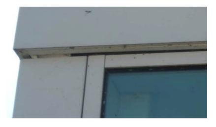
**La-Z-Boy Center** – It appears there is a void within the exterior aluminum, curtain wall assembly allowing the environment to enter the interior.
