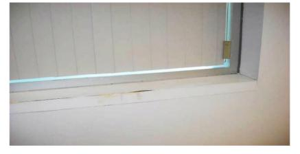
**Whitman Center** – water infiltration along exterior wall has caused deterioration of the plastic-laminated windowsills.
