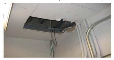
Whitman Center - breach in fire-rated ceiling assembly.
