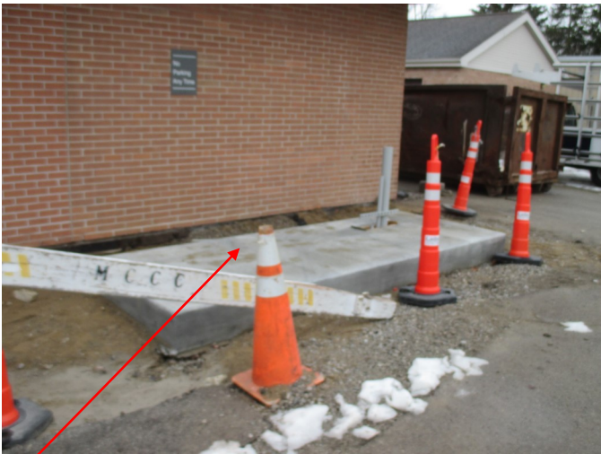
The top-left photo shows one of the six new pads that were created for the future generators. The one featured in this photo is outside the southwest corner of West Tech (#1). This generator will service E/W Tech and will eventually be screened by a new block/brick wall.
