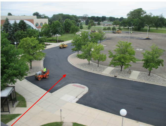
The top-left photo shows the paving contractor placing the base layer of asphalt in Parking Lot 2 near the bus stop in between the La-Z-Boy Centers and the Life Sciences Building.
