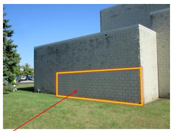
In the top-left photo the highlighted region shows the stark contrast where the existing split-face masonry block has been washed as opposed to rest of the wall where the wall is still soiled. The contractor performing the work for this project is using a combination of an environmentally-friendly process that uses a detergent and warm water along with a pressure wash to clean the façade.
