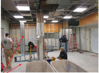
In the top-left photo you can see the extent of the renovation of the old cafeteria serving area over to the new micro-market. The area was stripped down to bare studs and floor slab. New walls were constructed as necessary to house coolers, racks, cabinetry, etc. Additionally, the old ceiling and lighting was removed and replaced with new tile and LED lights.
