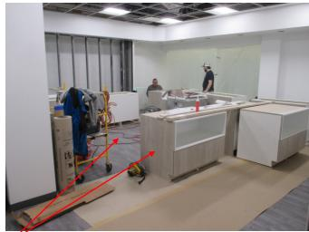
In the top-right photo one can see the progress of the renovation. The new walls are finished as well as the new floor tile has been installed. Here the contractors are also beginning the installation of the new cabinetry that house supplies (along the east wall) and supplies/microwaves (west wall).
