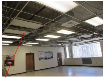
The top-left photo shows the very beginning of the demolition of the ceilings in one of the classrooms. Each of the classrooms will receive new paint and wall base, new flooring, new ceiling grid/tile and LED lighting, new A/V systems, and new furniture.
