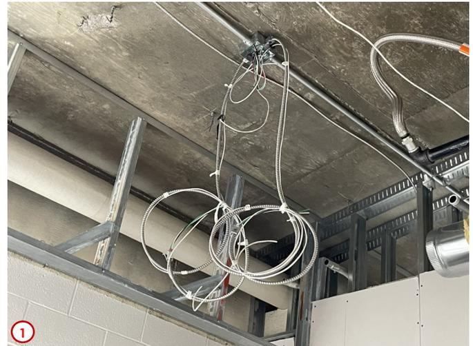
Photo #1 features one of the many instances where the wires have been pulled and whips ready to connect to the future lights in the ceiling in the H/SS Division Office Suite.
