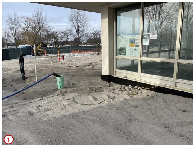
Photos 1 and 2 shows the final step completed for the targeted basement waterproofing as the area has been backfilled.
