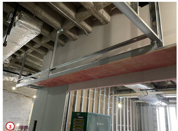
Photo #4 shows some of the need supports for future countertops, shelving systems, etc. now in place. With all of this infrastructure in place the wallboard can be finished.
