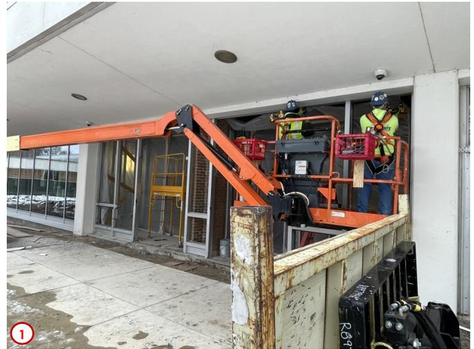
Photo #1 was taken earlier in the week and shows the glazing contractors installing some of the new curtain wall frames at the old west entrance of the Library. A row of offices now line this wall and so the old entry door system was removed.
