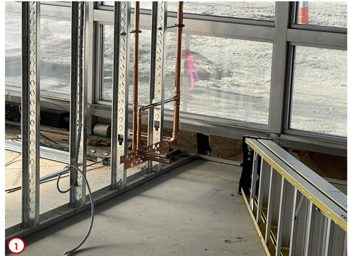
Photo #1 was taken in the area that will become the new east vestibule in the main corridor on the first floor. Here you can see more of the mechanical infrastructure now installed. Featured is the in-wall hydronic piping that will supply the unit cabinet heater that will provide supplemental heat.
