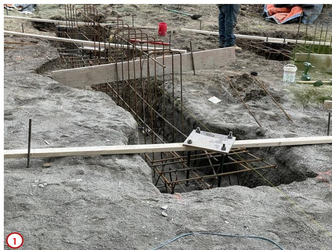
Photo #1 was taken outside the future east entrance on the first floor, and shows the trench excavated for the foundation system for the new canopy that will be installed in this area. You can also see the steel reinforcing bars and location for the anchor bolts will allow the structural steel to anchor to the foundation.
