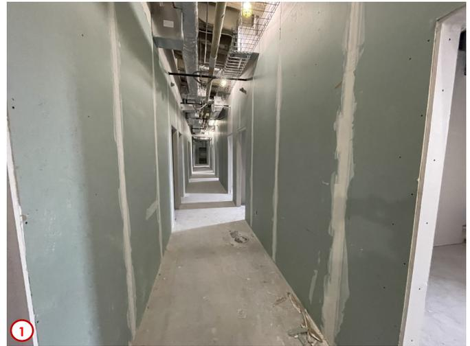
Photo #1 highlights the progress of the finishing of the wallboard on the second floor. The area featured in this photo is the corridor in the new H/SS Division Office Suite. Here you can see the joints for the wallboard being taped and mudded. Next week the contractors will start to sand the joints so that later the wallboard can receive its coats of primer and paint.
