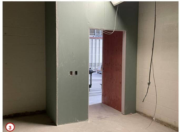
Photo #4 shows an area on the second floor in the existing janitor's closet where some additional demolition work was recently completed. Here the wall was opened so some conduit can be run from the mechanical penthouse above down through and eventually into the basement. These conduits will house everything from new electrical wiring to communication cabling. A new wall will be built out which will also enclose the recently installed conduit in the foreground.
