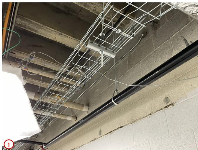
Like the 2nd and 1st floors the basement is now having a lot of its above ceiling infrastructure being installed. For example, in Photo #1 one can see not only the aforementioned fire sprinkler main trunk lines now in place, but now next to the cable tray is in that will hold all of the new data cabling that will feed all the classrooms, offices, etc. in the area with network connections stemming from the main server in the southwest corner of the basement.
