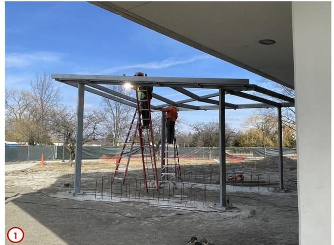
Photo #1 highlights the beginnings of the erection of the structural framing system for the new entrance canopy on the west side of the building. Here you can see the contractors welding some of the smaller cross members to each other to solidify the integrity of the entire structure.
