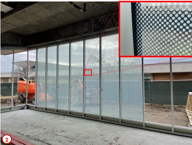
Photo #3 was taken later in the week and shows all of the glazing panels installed for the northwest addition. Now the contractors will focus on replacing and/or repairing the soffit adjacent to the additions to help weather-proof the envelop of the building. This addition will house huddle rooms for use by staff and students in the Library.
