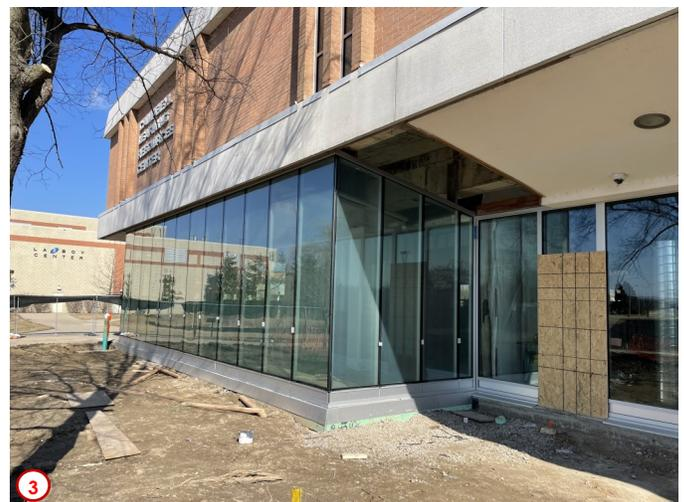
Photo #4 was taken on the same day as Photo #3 and shows the now completed curtain wall system for the southeast addition (the larger of the two additions). This addition will house two spaces: a classroom, and a computer lab. The framing of the interior walls for these two new spaces can now begin since the curtain walls are now complete.
