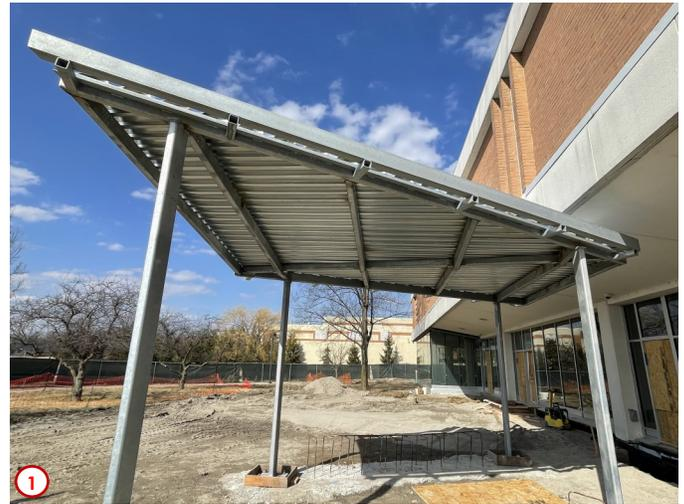
Photo #1 highlights the progress of the work needed to complete the new western entrance canopy. The structural steel for both canopies is now in place, and therefore the contractors can begin the process of installing the framing which will then lead to the finishes being installed.
