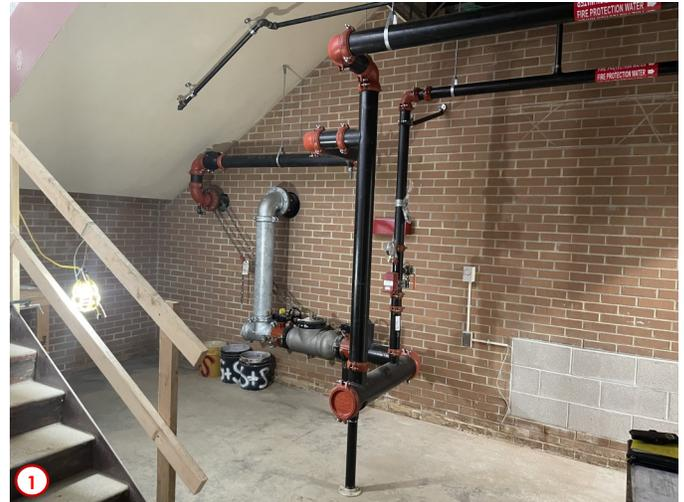
Photo #1 shows the progress of the installation of the new fire riser in basement near the west stair tower. Once completed the fire-rated partition that will help separate the new room in which this unit will reside will start being constructed.
