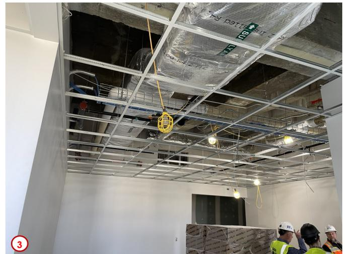
Photo #4 was taken of one of the many instances where more of the low-voltage cabling has been pulled and ready for termination. The instance shown happens to be in what is the Adjunct Faculty Office on the second floor in the H/SS Division Office. This data cabling will eventually allow cables to be connected through furniture systems that will be populated by computers for staff use.
