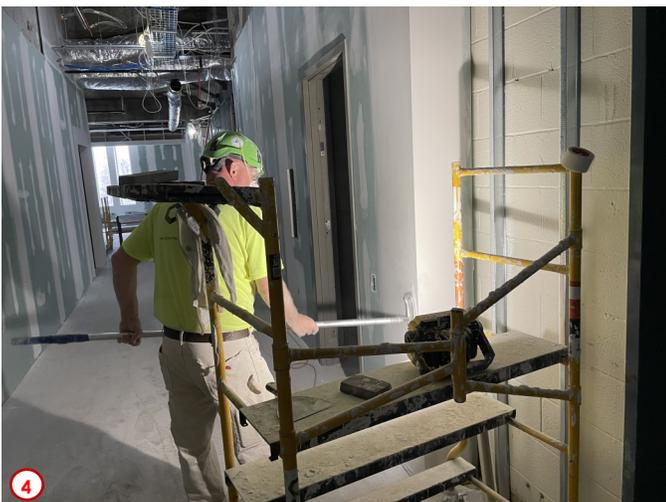
Photo #4 shows one of the many interior contractors sanding one of the new joints in the wallboard near the existing elevator door on the second floor. After all the seams, joints, corners, etc. are taped and mudded all that has to be properly sanded before the painters can come in and apply the multiple layers of primer and finish paint.
