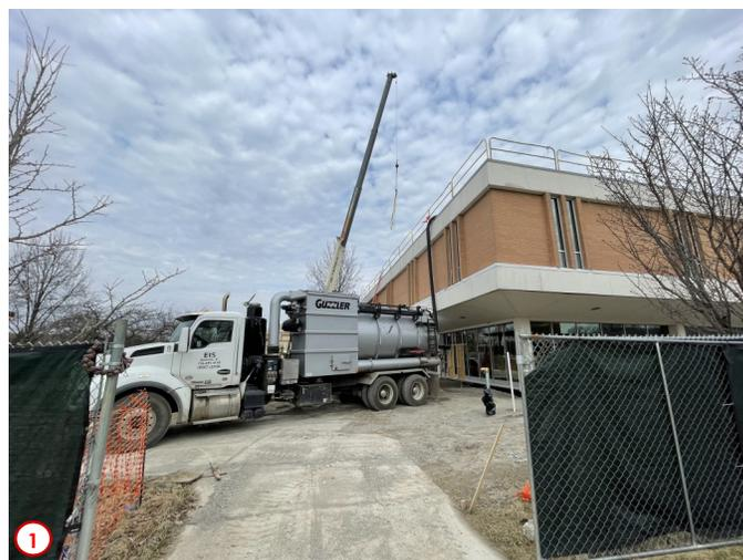
Photo #1 features the vacuum truck that was used to remove the existing stone ballast from the roof. In the background you can see the crane that has been set up to convey the new roof materials and needed installation equipment.
