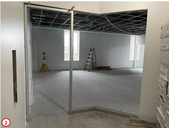
Photo #1 was taken inside one of the existing classrooms that are being refurbished as part of the overall project. Here you can see the new suspended ceiling grid system now in place and ready for the electricians to install the new LED light fixtures.
