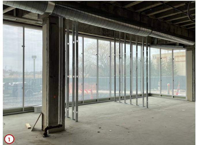
Photo #1 shows the progress of the installation of the rough framing in the northwest addition on the first floor. Here you can see the partition walls that will separate the future huddle rooms off of the Library being constructed.
