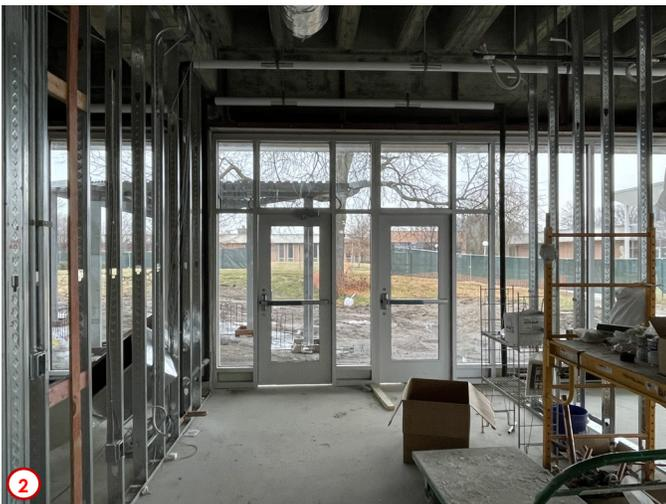
Photo #3 highlights the progress of more of the installation of some new rough framing being installed on the first floor. Here one can see some furring channels that have been installed over the existing masonry walls that will later receive a later of wallboard and be finished.
