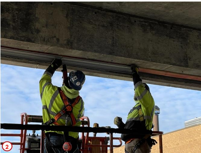
Photo #2 was taken in the area of the southeast addition to the first floor that will eventually be a classroom and computer lab. Here you can see the glazing contractors installing the top track for the curtain wall system in this area.
