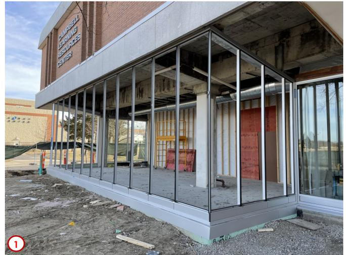
Photo #1 shows all of the curtain wall framing now installed for the northwest addition off of the future Library. In the next few weeks all of the openings will be infilled with glass panels to finish the exterior envelope of the first floor.
