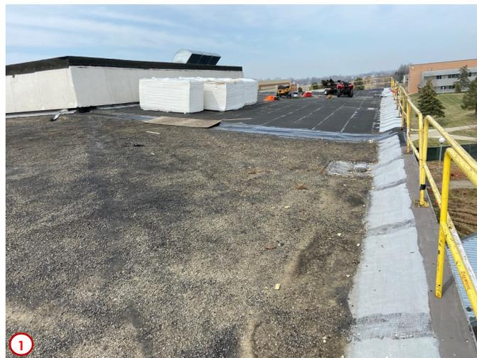
Photo #1 was taken along the east side of the lower portion of the roof. Here you can see an example of how the roofing contractors have been working in smaller sections. This way they can get the work accomplished even with the extra rainy weather we have been experiencing lately, and by doing this they are able to keep the interior of the building dry.
