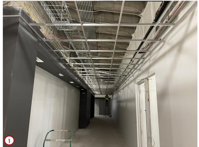
Photo #1 shows the now completed grid system for the suspended acoustical ceiling tile in the new north corridor on the second floor. With this grid in place several infrastructure items can be installed such as the sprinkler heads, air diffusers and return grilles, occupancy sensors, and light fixtures.
