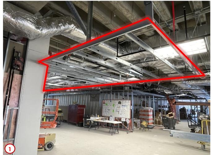
Photo #1 shows the light-gauge metal framing (highlighted for your reference) now installed for the bulkhead that will be above the reference desk area in the library space. This framing will eventually be clad in a panelized wood veneer system.
