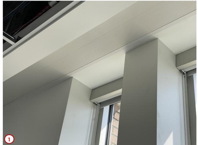
Photo #1 was taken in the staff lounge in the H/SS Division Office Suite looking at one of the grouping of windows. This photo features two new recently installed items the first being the new shades for the windows, and the radiant heat panels. The radiant heat panels are set into the soffit between the existing exterior wall and the new bulkhead, and help supplement for any heat loss caused by the windows.
