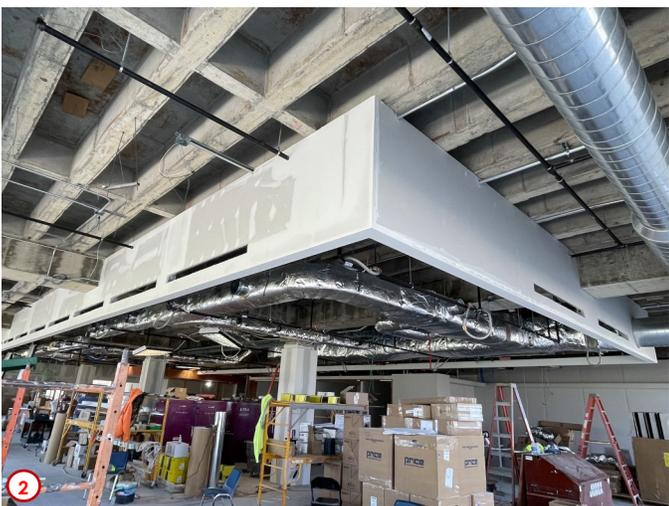
Photo #3 features one of the many new supplemental heating units now installed on the first floor. The unit featured in this photo is located at first floor landing in the east stair tower, and helps maintain the proper temperatures in this area due to any heat loss caused by the building occupants entering or exiting the building.
