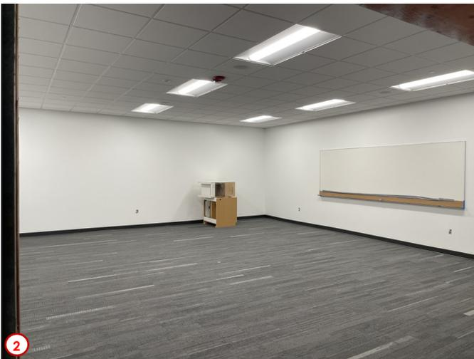
Photo #2 was taken in the classroom near the H/SS Division Office Suite, and shows the current status of most of the classrooms on the second floor, and that is their ceiling has been padded out (or received it's tile) and the carpet planks are now installed. The rubber wall base has also been installed soon this room will be ready for furniture once the new teaching station has been installed.
