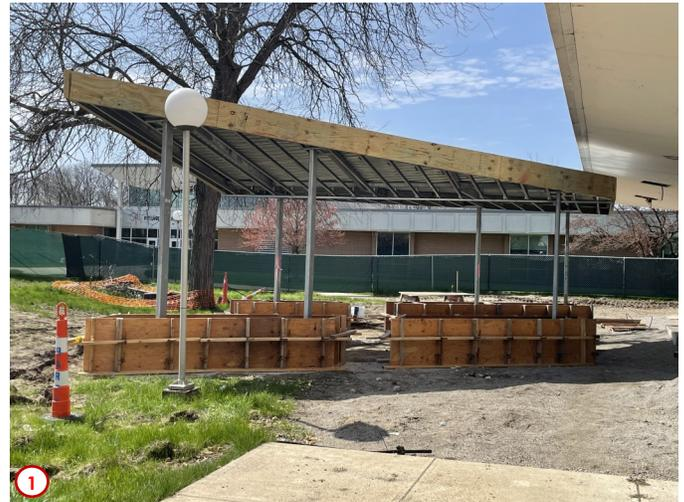
Photo #1 highlights the progress of the work on the new east entrance canopy. Here you can see more of the rough framing has been completed, and the formwork is in so that the concrete for the associated seating walls can be placed. This same process has been started for the new canopy on the west side of the building as well.
