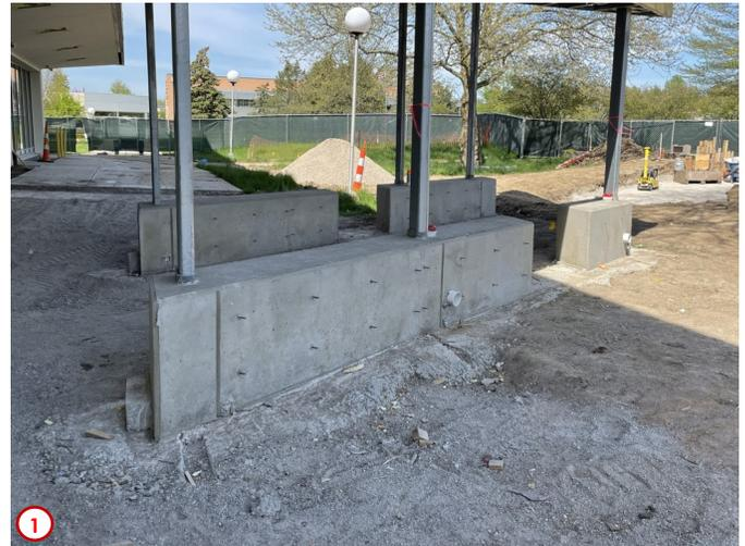
Photo #1 was taken outside at the new east entrance canopy. In the background one can see the landscaping work needed happening to install the new sidewalk that will connect the new east entrance to the central mall of campus for enhanced pedestrian traffic. In the foreground you can see that the concrete for the seating walls was placed this past week and await finishing.
