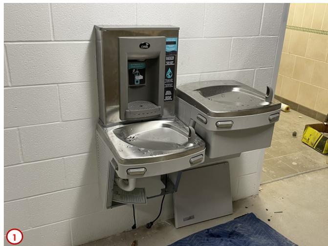
Photo #1 features one of the several new electric water coolers that are being installed throughout the building. Unlike the old units these are both ADA compliant and feature a bottle filling station which is a new standard that is being implemented campus-wide.
