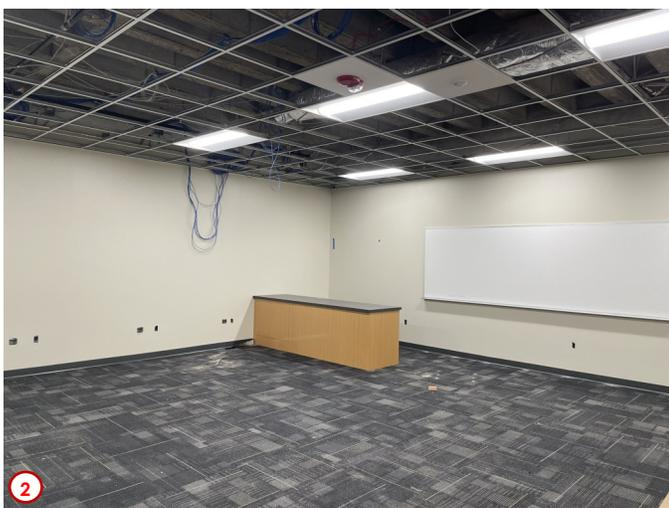
Photo #2 was taken in what will be the designated computer lab in the basement and shows nearly all of the finishes complete minus the ceiling tile. Also featured in the photo is the new marker board and teaching station. Once the ceiling is complete the only remaining items left to be installed in this room will be all of the instructional A/V equipment and the furniture.
