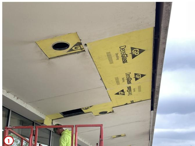
Photo #1 was taken outside the northeast corner of the building. Highlighted in this photo is the work being done to repair the soffit under the second floor where it had to be cut open to run some new plumbing lines. Once the substrate is complete plasterers will come in and install a scratch coat and final coat of synthetic stucco to match existing. The entirety of the soffit will be painted once all the patches and new LED lighting fixtures are installed.
