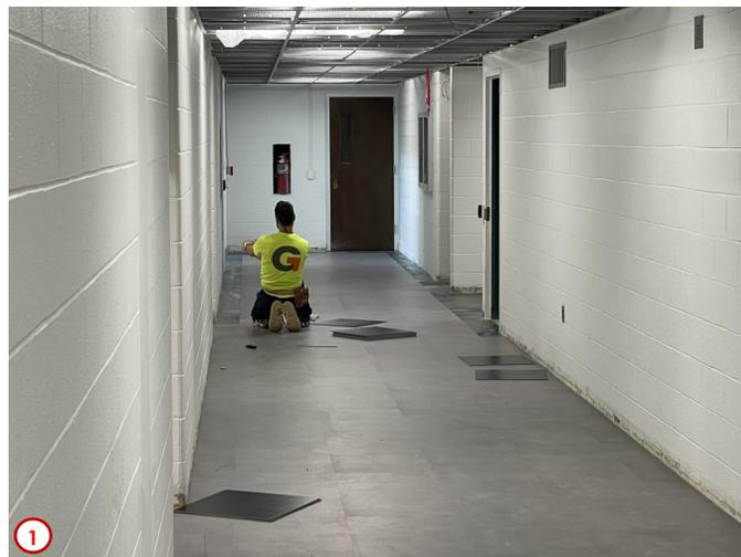
Photo #1 shows the flooring layers installing the LVT (luxury vinyl tile) in the basement corridors. Some of the main features we like about LVT over VCT (vinyl composition tile) is that it doesn't have to be stripped and waxed every year, and the color runs all the way through so scratches aren't as apparent. Therefore they are more robust and require less maintenance and therefore have a lower TCO (total cost of ownership).
