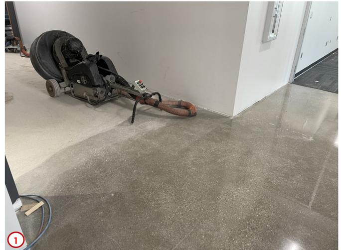
Photo #1 shows the results of the concrete polishing occurring on the second floor in the corridors. After the existing concrete is ground down to expose more of the aggregate it then is cleaned and polished to the level of gloss shown in this photo. This will be floor finish in the corridors on the first and second floor.
