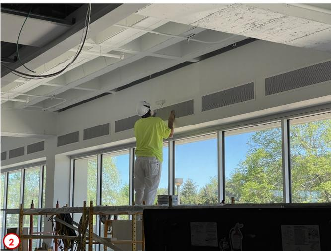
Photo #2 shows some of the many areas inside the library being finished. Here the bulkhead along the north perimeter wall is being primed and painted above the new air diffusers near an area where the ceiling will be left open to the structure above.
