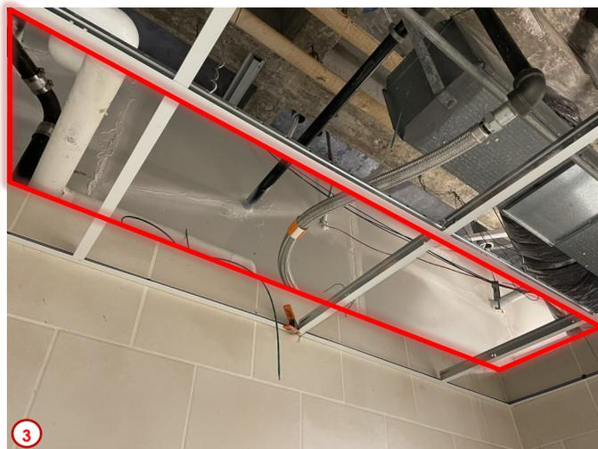
Photo #3 shows one of the small details that have been completed in the basement. Highlighted in the photo is a section of some additional framing, wallboard, and sound batt insulation (not shown) that was added to the top of the existing concrete block walls that divide the restrooms from each other and the adjacent corridor. This work will ensure better privacy and security in this area of the building.
