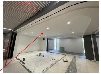
The top-right photo features the now finished ceiling at the top of the west stair tower. The wallboard has been finished and the new lighting is in place and working as designed.
