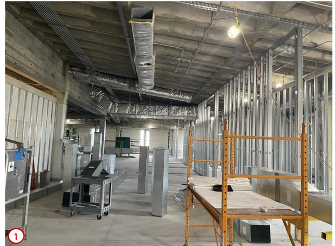
Photo #1 was taken in the area of the future H/SS Division Office Suite looking west. Along the right side you can see the stud walls forming that will be the faculty offices. On the left side you can see furring being applied to the existing masonry wall so that new wallboard can be installed. Then at the top you can see more of the existing duct-work has been insulated.
