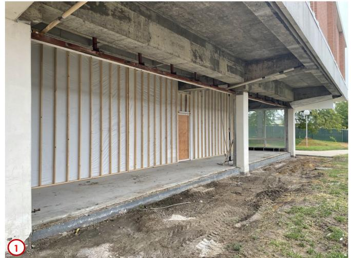
Photo #1 shows the now completed demolition of the old curtain wall system along the southeast portion of the first floor. In the next few weeks this area will be excavated so that the waterproofing system can be installed on exterior face of the basement wall. Once that is done the foundations for the addition in this area can be installed.
