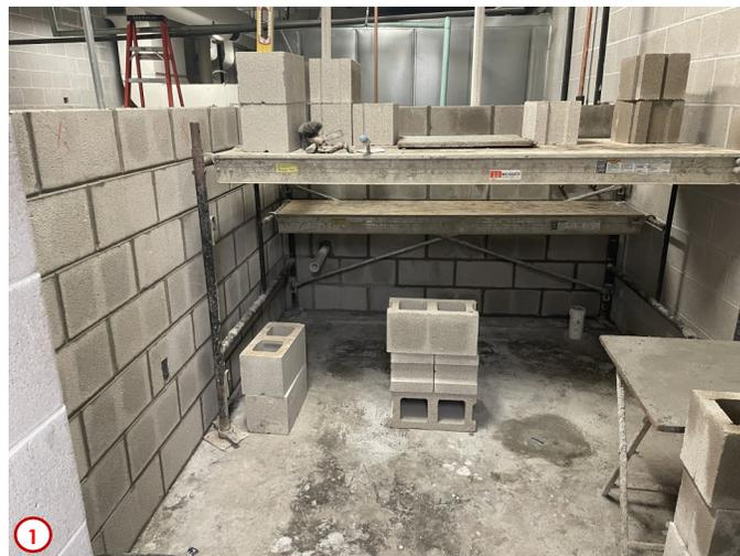
Photo #1 highlights the progress of the construction of the new janitorial closet in the basement of the CLRC. Again, the concrete for the floor slab has been placed and now the concrete block walls are being laid to fully enclose the space. You can see underneath the scaffolding the rough-ins for the future mop sink and oil separator along the east wall.
