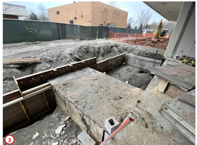
Photo #4 is another shot the formwork for the southeast addition on the first floor, but offers another perspective and provides a better idea of the size of this future space. The southeast addition is much larger than that which has already been started at the northwest corner of the building. This addition will house a classroom and computer lab when eventually completed.
