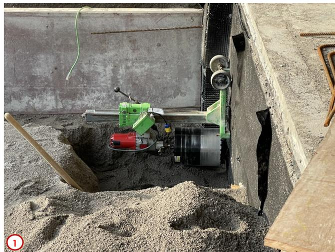
Photo #1 shows some work that is happening in conjunction with the basement waterproofing, and it is replacing some drain lines (both storm and sewer) that exit the building below grade and connect to their respective campus-wide underground utilities. The original pipes were breaking down and will be replaced with and hopefully longer lasting materials. In order to do this the basement walls had to core-drilled in order to allow for the newer and properly sized piping.
