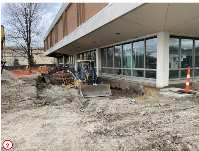
Photo #2 is off the last area along the southwest corner of the building where the targeted waterproofing is being finished. With this completing this will allow for the foundations for the canopies to go as well as the new entry to be installed in this area that will serve as the new "front door" off of Parking Lot 7.
