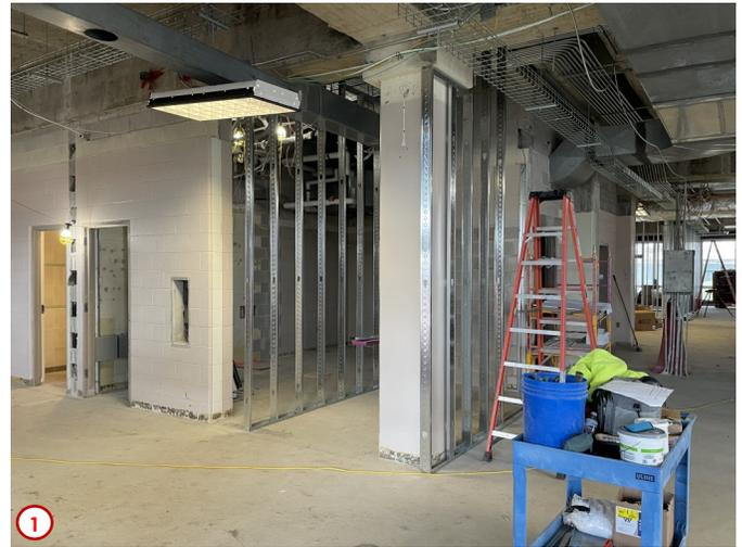
Photo #1 was taken from the area of the future west vestibule on the first floor looking at the area that will become the private room. This is yet another area that had rough framing installed as the contractors have made significant progress in getting all of the walls framed in for the entire first floor.
