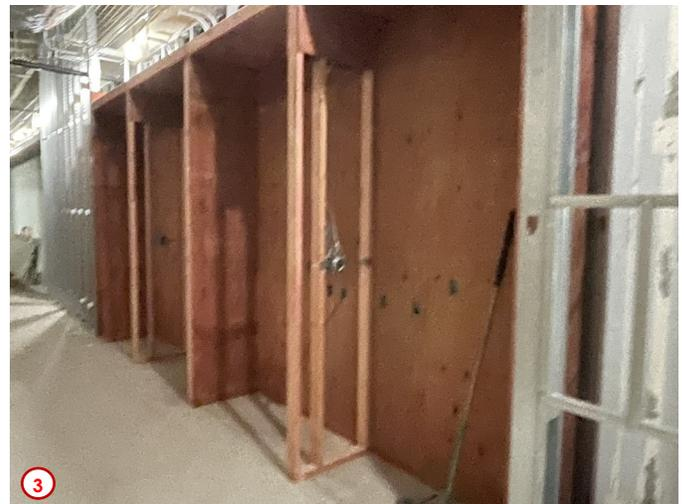
Photo #4 shows the progress of the installation of additional wallboard and framing in the east corridor. This corridor is existing and is receiving a wallboard finish on metal furring channels. This new finish will not only be more attractive than the existing masonry walls, but will also help with acoustical legacy items and will hopefully cut down dramatically on the echoes that used to plague this area.
