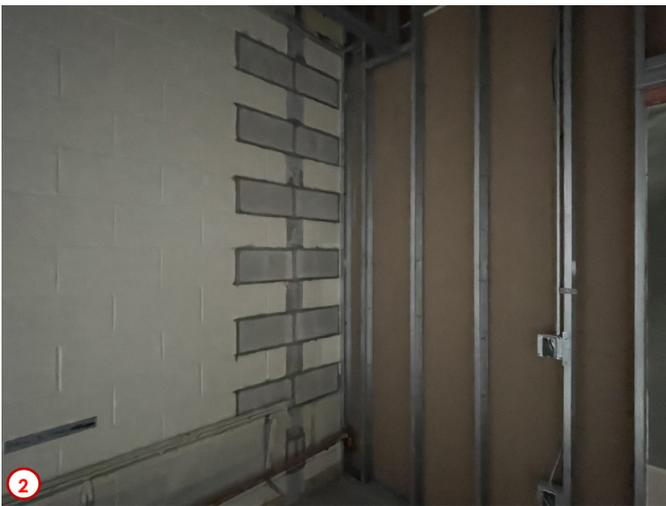
Photo #3 highlights the progress of the framing being done for the future single occupant study booths being constructed in the new north corridor between the classrooms and the H/SS Division Office Suite.
