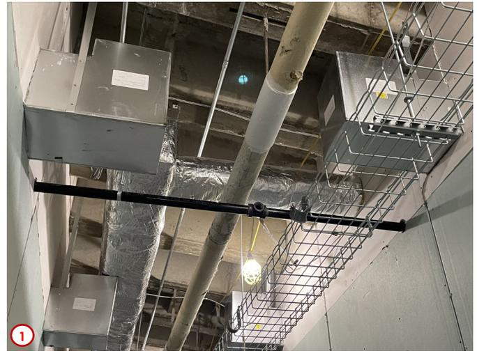
Photo #1 shows the progress of the installation of the fire sprinkler system on the second floor. Featured in this photo is a branch line running through the corridor in the H/SS Office Suite. The empty threaded connection will receive a down pipe that will terminate at one of the hundreds of sprinkler heads that will be eventually installed.
