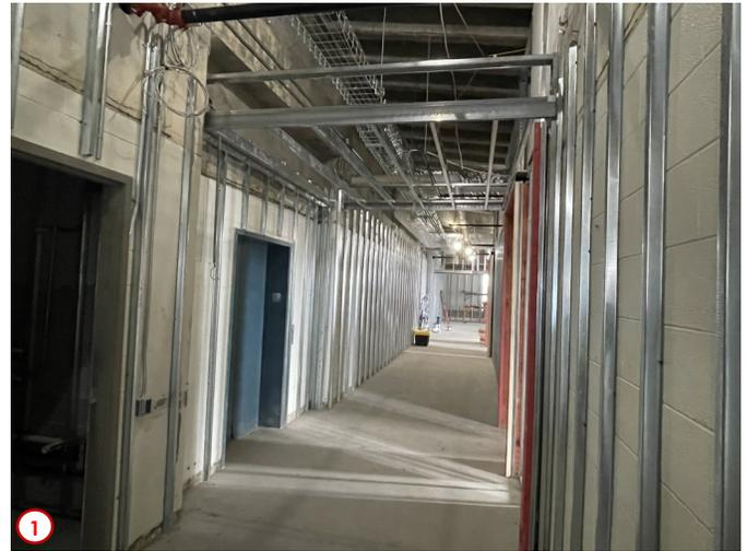
Photo #1 highlights the installation of some additional framing that is meant to help break up the south corridor, but more importantly mark the location of the elevator which will assist in wayfinding for the building occupants.
