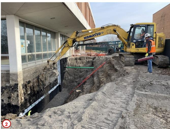
Photo #2 highlights part of the process of backfilling in around the basement walls. The backfilling is done in "lifts" and instead of placing back the old soil which was comprised of mostly clay and did not drain well the new fill is mostly crushed limestone that is compacted after being placed. This will serve as a good filtration system and provide a sturdy base for the new top soil and sidewalks that will be installed near the completion of the project in the spring.
