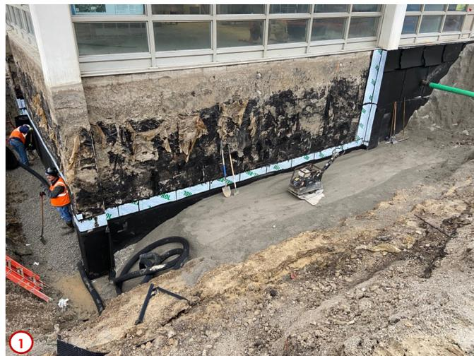
Photo #1 shows the last stretch of basement waterproofing being completed. Additional to the work for the waterproofing in this area to the building proper there will also be some new storm sewer work completed to provide better drainage for the area surround the CLRC.
