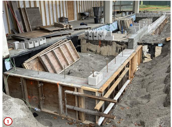
Photo #1 was taken earlier in the week and shows the foundation system concrete placed in the forms with the first of the concrete block being installed.
