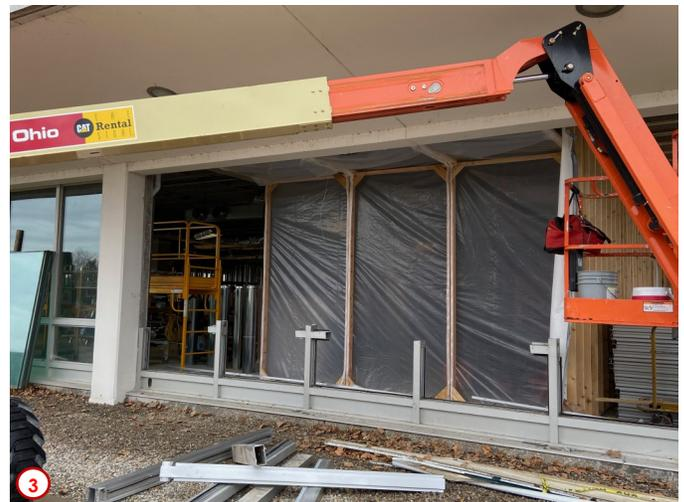
Photo #4 was taken later in the week in a similar location to that of Photo #3 and shows the first section of new curtain wall installed. The new curtain wall is on the right and the existing is on the left. This new curtain wall has a different look to it which will update the aesthetics of the exterior of the building, and is also much more energy efficient.
