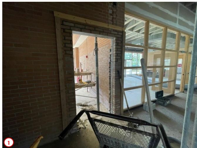
Photo #1 highlights the progress of the work at the first floor landing of the eastern stairwell. Both of the old double door openings have been filled in with cmu and existing brick, and then the new single door opening has been cut in and salvaged brick is being used to finish out the opening so the new door frame can be installed. This change was necessary to facilitate the new Library Staff Office Suite which will be partially located where the old main entrance to the space was located.
