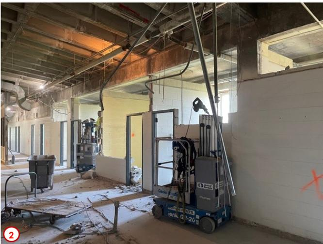
Photo #3 was taken later in the week after the previous two photos and shows the fact that all the walls in that area were removed and the debris cleaned up and properly disposed of. Soon new framing will be installed per the architect's plans.
