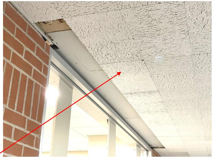
The top-right photo shows the installation of the new spline ceiling files that match the existing in the area.
