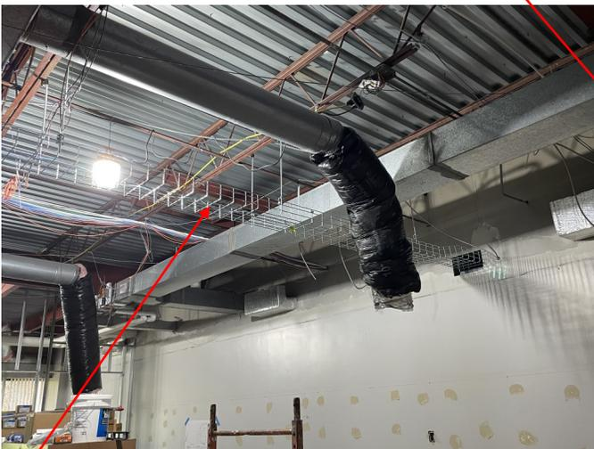
The bottom-left photo shows the remaining portion of the cable tray for this space now properly installed and ready to house future information systems communication lines. This cable tray connects across the corridor to the new set installed there and eventually terminates in the south IT Room.
