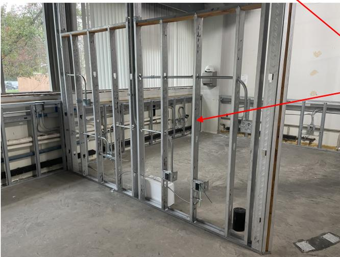
The bottom-left photo highlights the progress of the installation of the electrical infrastructure at the Student Government Room Office. Once all of this work is complete wallboard can be installed and finished on both sides of the wall.
