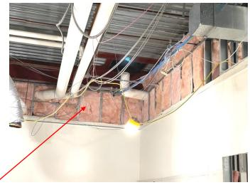
The top-right photo shows some of the measures being taken to help provide acoustical separation for the new HR Office Suite. Here you can see that batt insulation was added to the underside of the roof deck above which was then covered by a layer of wallboard which should help stop sound pollution.
