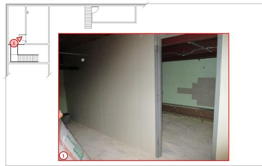
Photo #1 shows the progress of the work in the IT Room on the 2nd Floor of the Physical Plant. The new wall separating the new IT Room from the new dedicated mezzanine area has been constructed, and the door frame installed. Next up for this area is the insulation for the exterior walls and the new steel access stairs.
