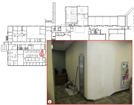
Photo #2 is in the Administration Building near the Admissions Office where the two old doors have been removed and covered. The only parts left are to paint the walls and install new wall base.
