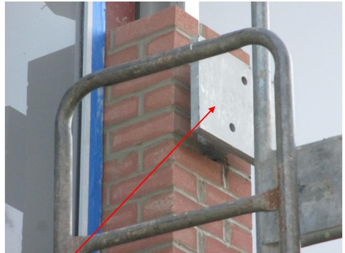
The top-right photo shows some of the new brick work around the new anchor plates for the new metal sunshade system to be installed later.
