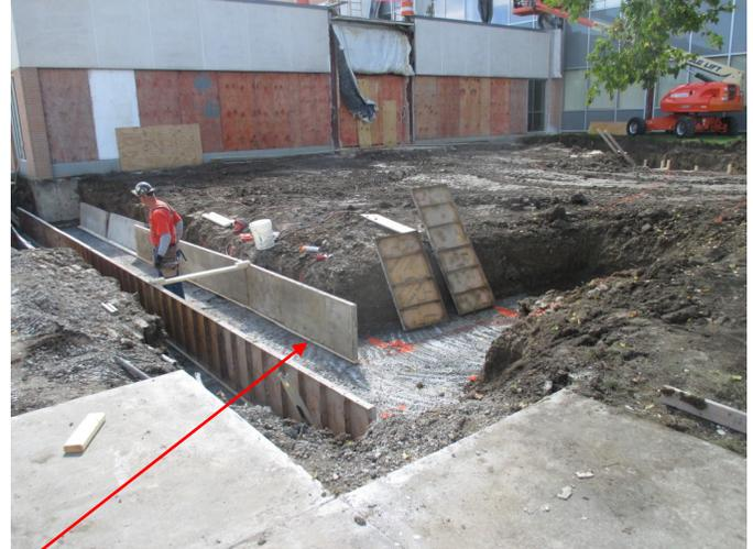
The top two photos show some of the formwork being installed for the foundations for the addition. The contractor has poured a "mud mat" for the forms to sit on due to the wet soil conditions.
