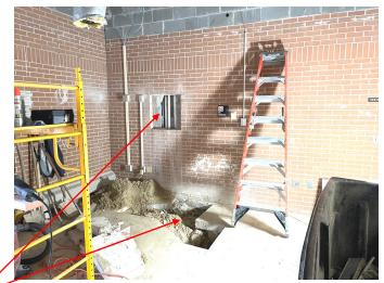
The top-right photo shows the contractors having exposed areas of the existing wall and floor slab so as to again access to existing plumbing infrastructure. Having access to these systems will allow the new plumbing to be connected into existing systems.
