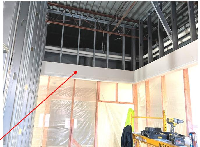
The top-right photo shows the new bulkhead in place that will help transition the new ceiling in this area into the existing. This bulkhead is needed because the existing spline ceiling tile system is no longer being produced or used and now a suspended acoustical tile ceiling system will be installed instead.
