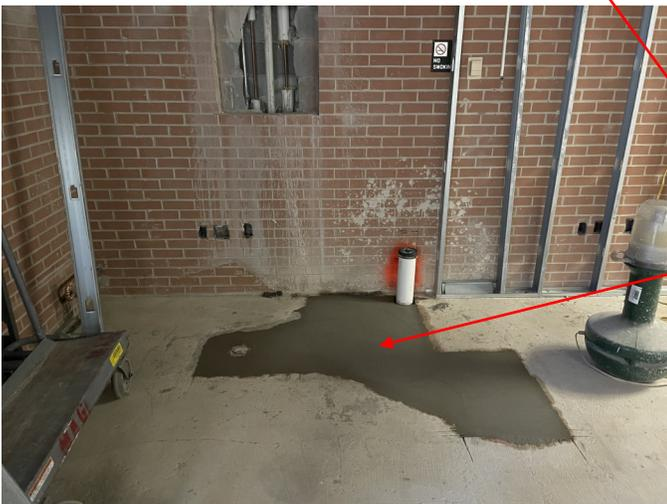
The bottom-left photo shows the new patch installed in the floor slab, and once cured will be ready to receive the new ceiling tile floor finish slated for this room.
