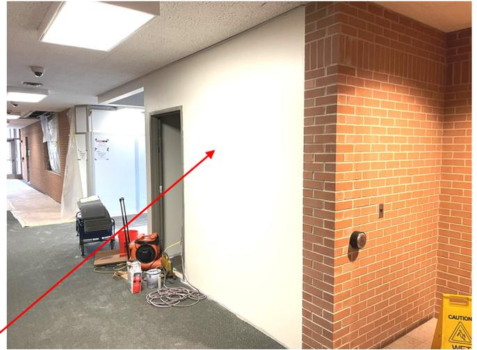
The top-right photo shows the exterior face of private room with the wallboard finished and painted. The door frame has been painted to match others in the area. Soon the ceiling systems in both spaces will be installed along with the doors.
